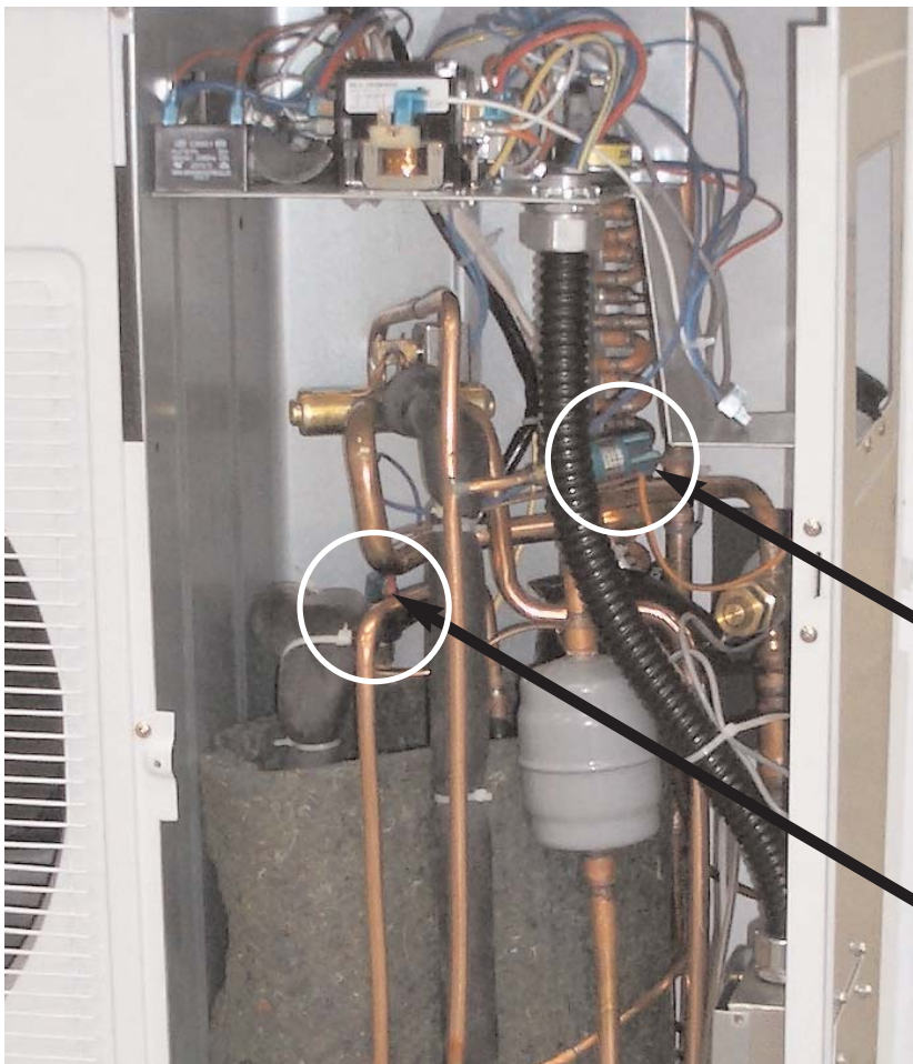
High Pressure Switch (green) open 450 PSi closed 250 PSi
