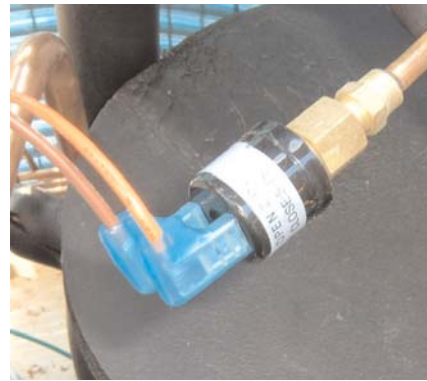
Low Pressure Switch (black) open 25 PSi closed 50 PSi
