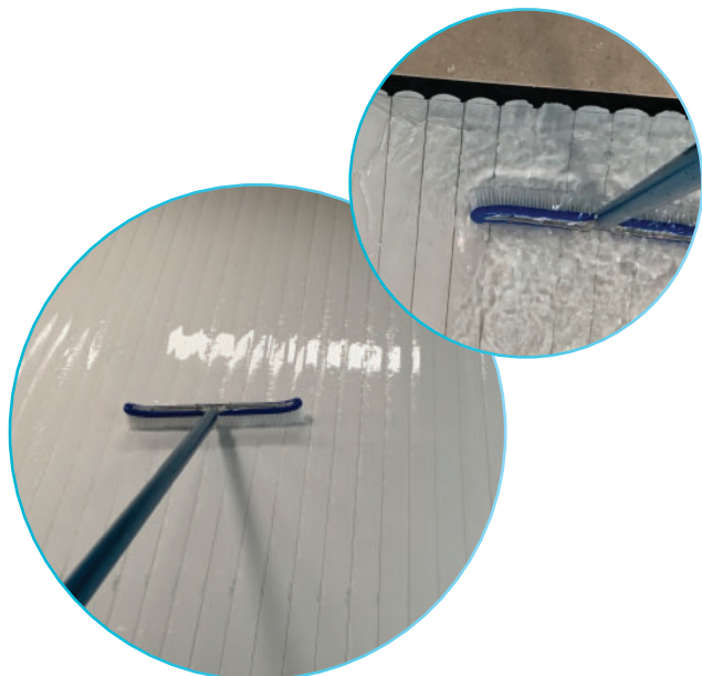
USE POOL BRUSH TO REMOVE REMAINING DEPOSITS
