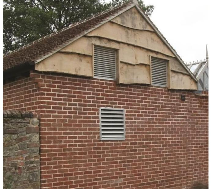
Simple test! To find out if the air supply is adequate, open the shed door while the pump is in operation. If the door moves, this means that there is a difference between the inside and outside pressure. Therefore, the shed is too airtight and a greater supply of air is required. If there is an inadequate supply of air, the heat pump could freeze, even with high outdoor temperatures!
