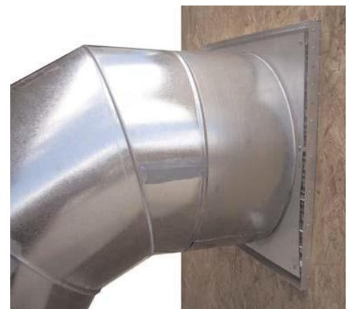
**STEP 6** Apply self-adhesive fixing foam to the outside edge of the spigot. There is no need to fix the spigot to the fan grille.
